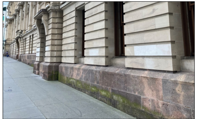
Brisbane Tuff plinth foundation, Treasury Building, Queen Street, Brisbane.
