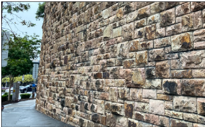
Brisbane Tuff retaining wall, Ann Street, Brisbane.
