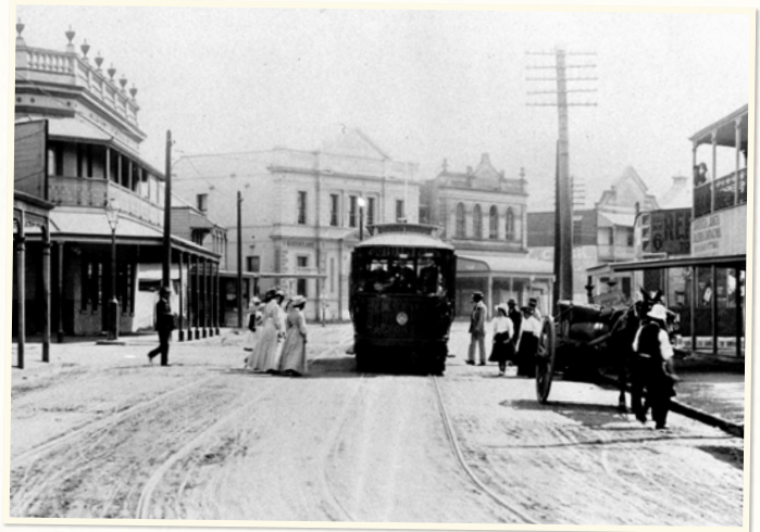
Albion Corner, 1909, State Library of Queensland, Negative No. 47139
