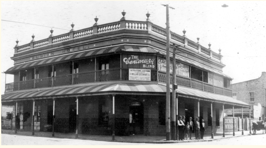
Albion Hotel on Sandgate Road, Albion, ca 1929, State Library of Queensland, Negative No. 1901
