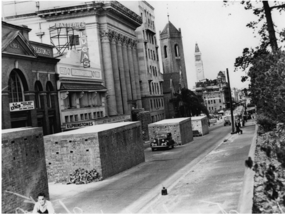
Air raid shelters with solid brick walls were called pillboxes because of their similar appearance to boxes holding medical pills. Ann Street, Brisbane, 1942 (State Library of Queensland)
