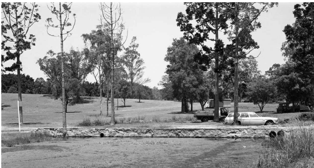
Figure 10 Dead and dying Kauri Pines behind the wetland weir in 1976.
