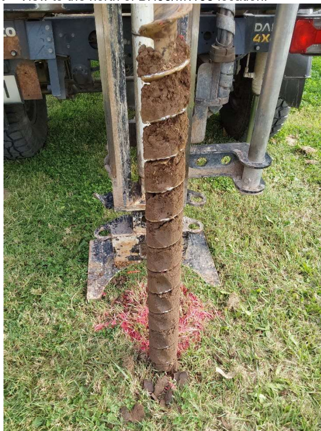
Photo 8: Secret Forest – BH03 surface to 1m BGL silty clay soil.
