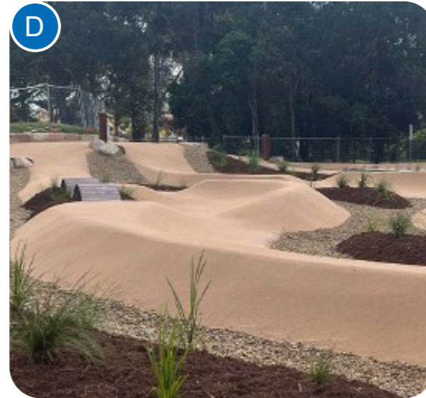
Berm Berm features are a fundamental component of a skills park, designed to help riders develop confidence and control when cornering at speed.
