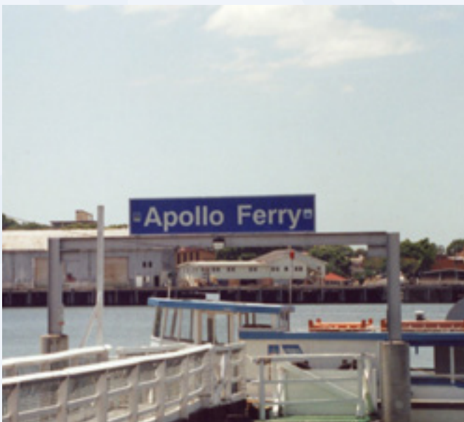
Apollo Road ferry terminal (1994)
