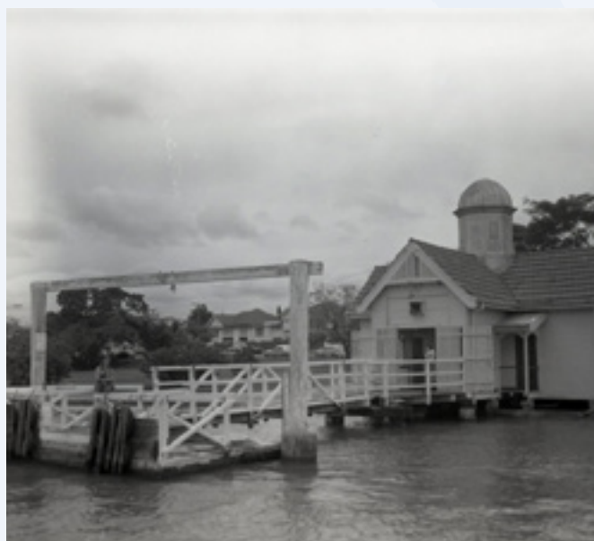
Hawthorne ferry terminal (1978)
