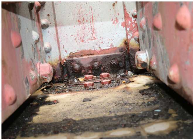
Box gantry rail bolt corrosion
