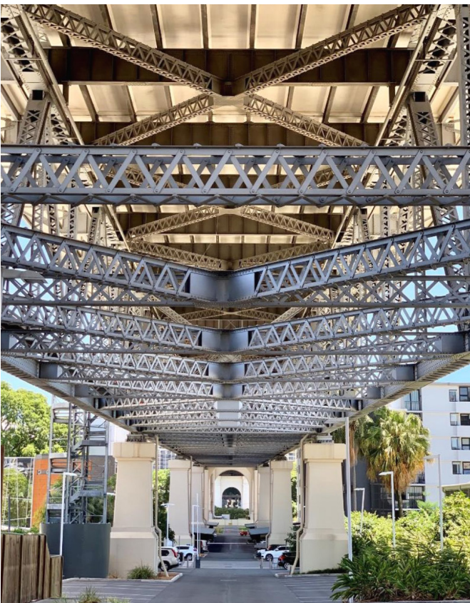
Steel frame of the Story Bridge
