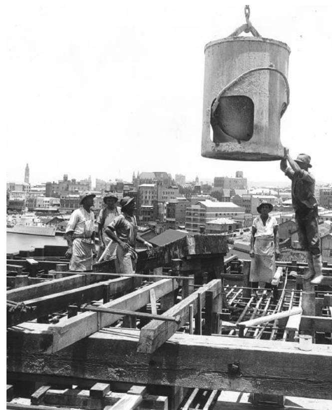
Concreting works on the Story Bridge - 1936
