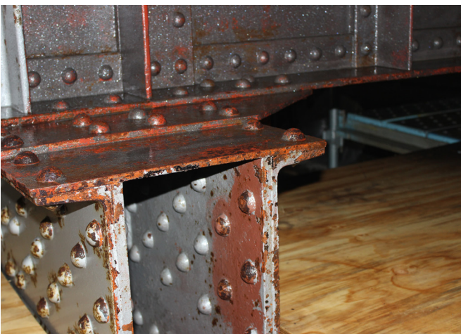
Box gantry rail bolt corrosion
