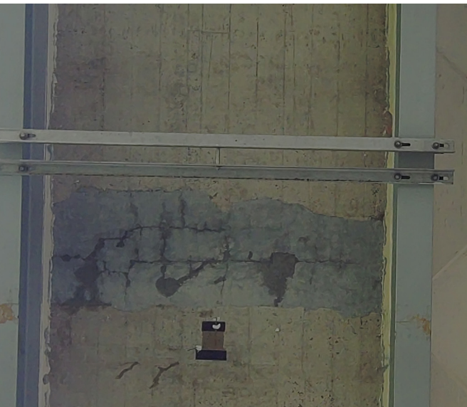
Water damage and concrete deterioration
