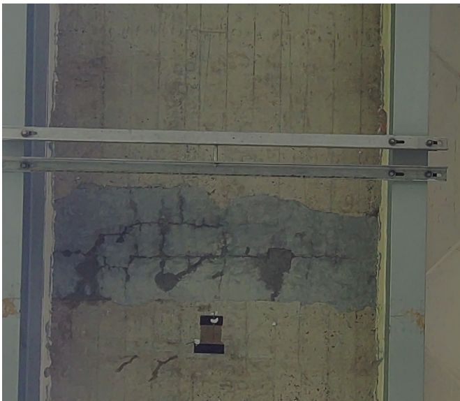
Water damage and concrete deterioration
