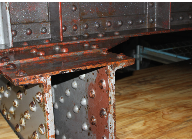
Box gantry rail bolt corrosion
