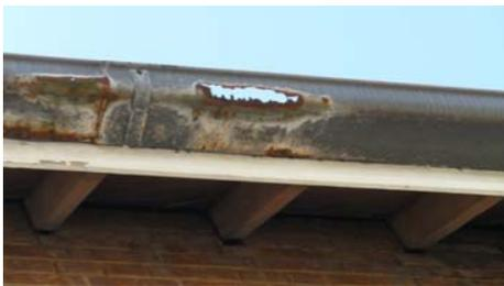
*Gutter deterioration due to 'drip spot' corrosion*
