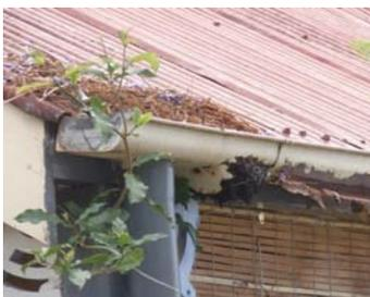
*Accelerated gutter deterioration due to lack of maintenance*
