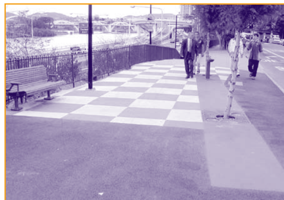
Figure h The use of different footpath patterns and colours is used in this example to highlight change of environment for cyclists and pedestrians.
