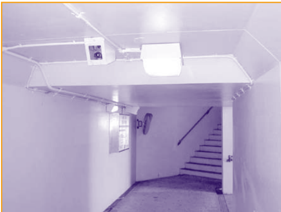
Figure s Risks associated with predictable routes such as underpasses can be alleviated with generous path width, use of surveillance technology, and the presentation of excellent levels of lighting, light coloured walls and signage
