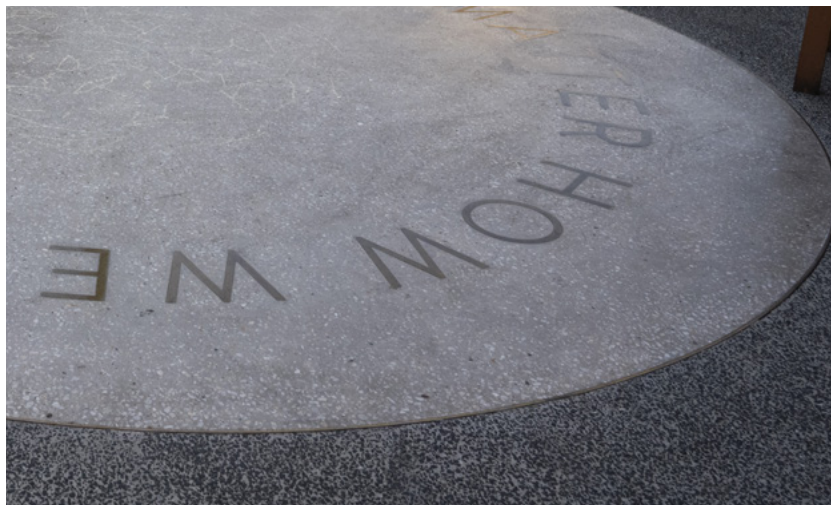
Example of honed-finish concrete (for plaza core) next to exposed-aggregate concrete finish (for around the plaza core)
